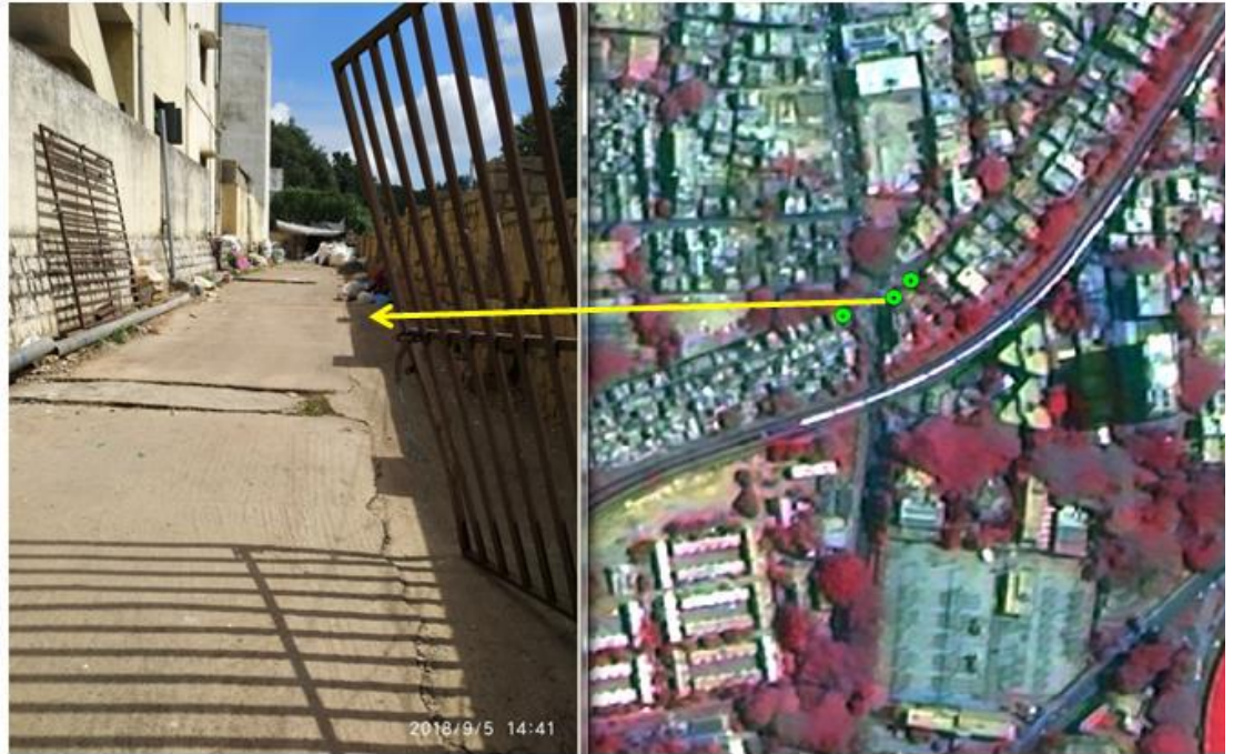
Covered drain in Sheshadripuram
